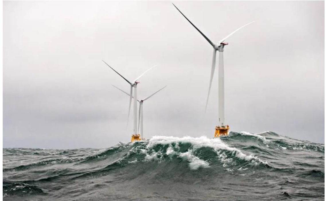
Block Island Wind Farm. Credit: Dennis Schroeder/NREL/flickr/CC BY-NC-ND 2.0
