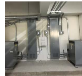
transformer & subpanels
