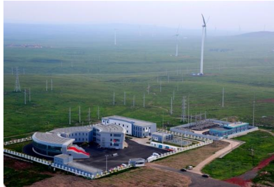
Zhangbei wind power test base, Hebei
